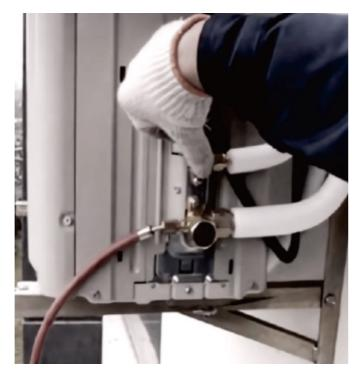
During the installation of air conditioner, carefully bend the pipe so as to avoid fracture, which may lead to the difficulty of sealing the cover plate.
