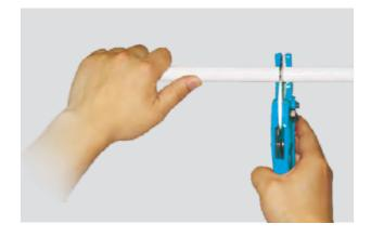
Cut the pipe vertically and precisely with a pipe cutter.
